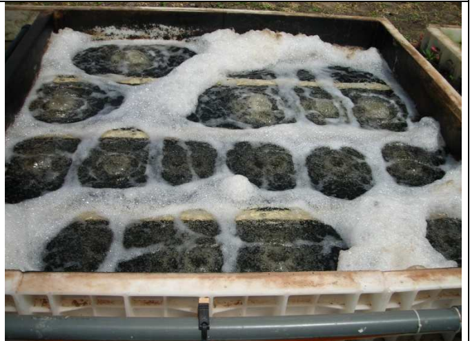
Jupiter 75 under installation in the onsite built concrete tanks
