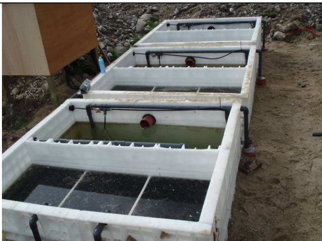
3 step Jupiter 25 system. To achieve the required cleaning, a 3 chamber Jupiter system is required.
