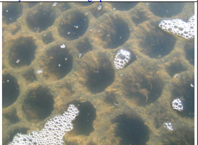
The bacteriological growth on the BioBlocks. The construction of the BioBlocks guarantee that the system does not clog up.
